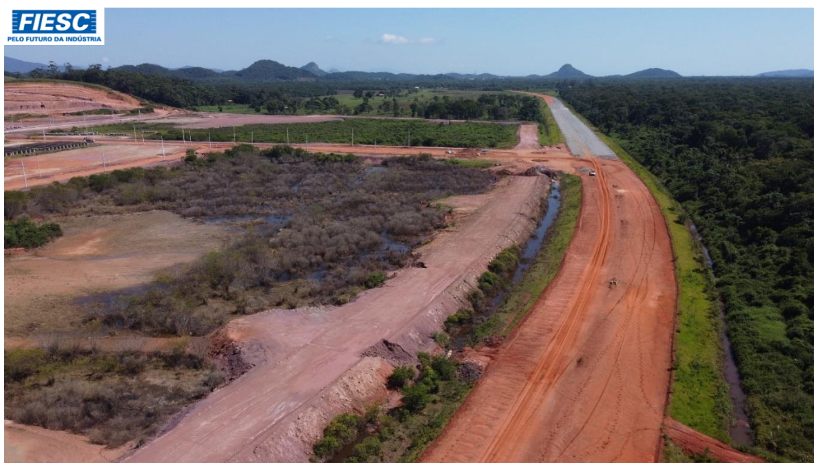
6: OUTRA VISTA DO SEGMENTO NO Km 9,0
